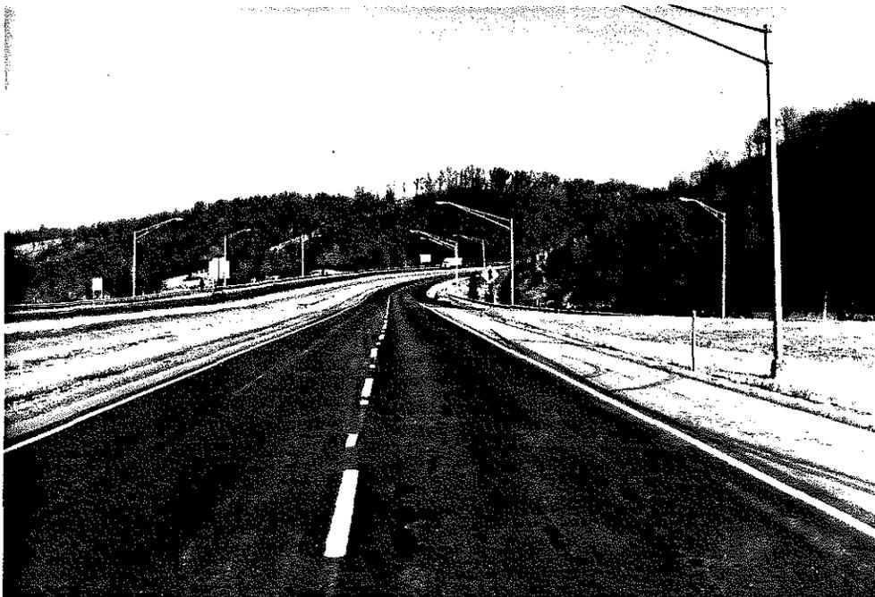
Figure 2. Two-Degree Curve.
