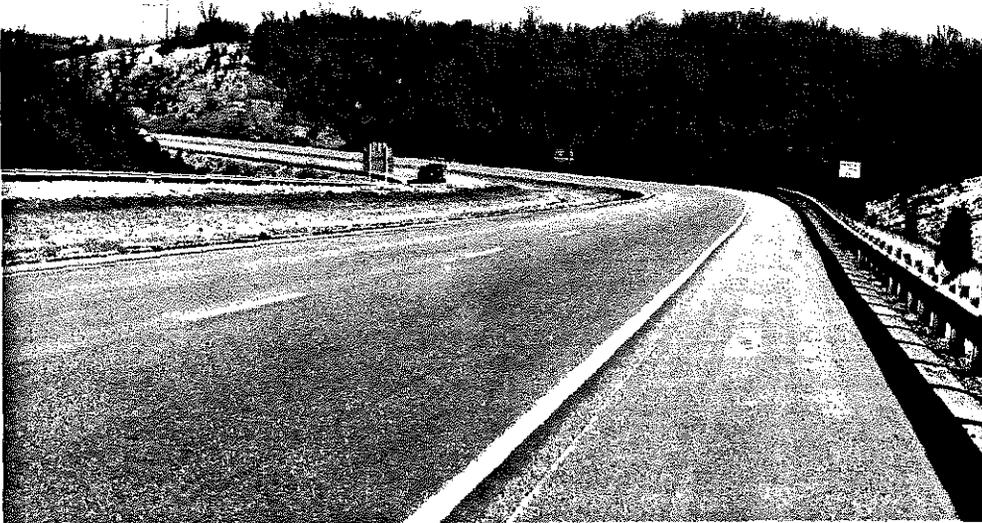
Figure 4. Four-Degree Curve.
