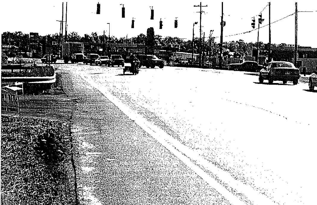
Figure 10: Lane Drop on KY 44 (Looking East)
