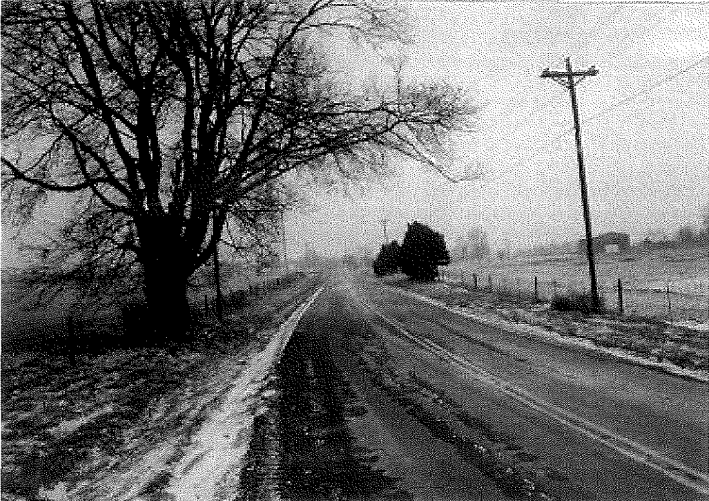
Figure 6: Clear Zone Limitations KY 101 North of Smith's Grove South of US 31W
