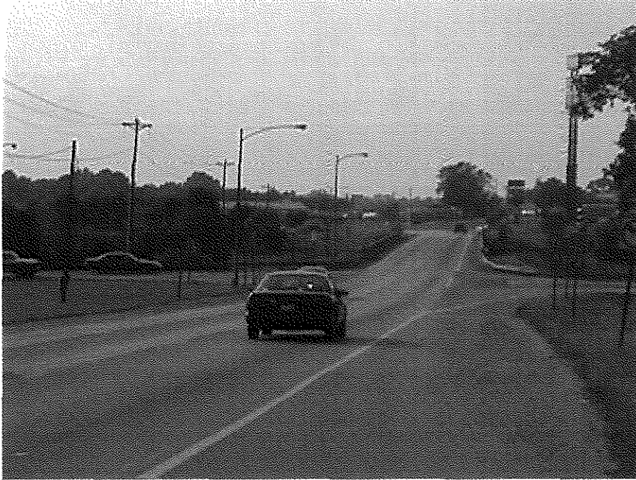
Figure 7: Northbound KY 153 at I-71 Interchange
