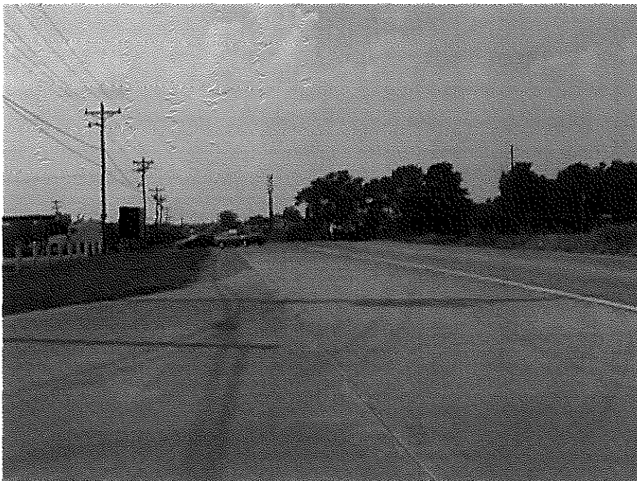
Figure 6: Northbound View of KY 153
